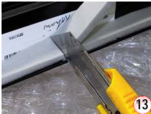
For sealing compound use: 1). Butyl Rubber Tape. 2). Double sided or one sided foam tape. 3). 100% silicone rubber sealant. 4). A suitable combination of the above.
