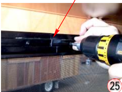
Start with the end screws and the clamping joint at the top of the window.
