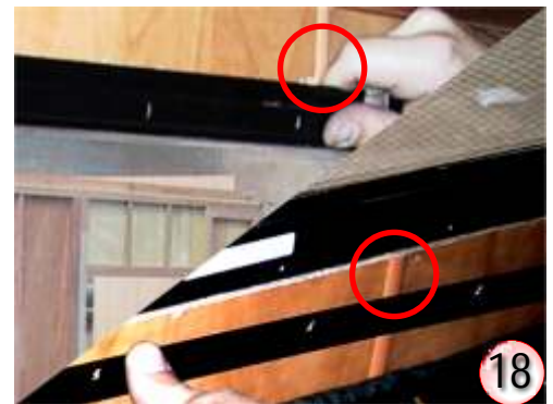
This T section of plastic extrusion may need to be cut out for the clamping to be positioned flat against the plywood.
