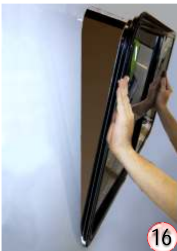
With the bottom of the window in place, gently push the top of the window in position in the opening.
