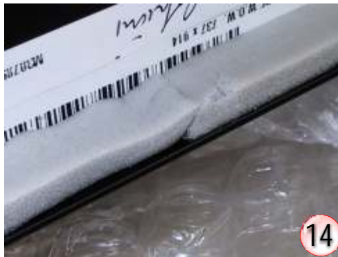
Apply Sealing Compound (in this case foam tape) all the way around the flange. Mid-Bottom of the window is a suitable starting point. Take particular care around the four radius corner. Cut off tape end at the starting point to form a continuous seal. Join foam tape, cleanly, as above.
