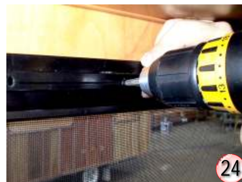
Install clamping in existing holes with a: No. 6 PAN HEAD - 12 mm long PHILLIPS screw. Stainless Steel or No. 6 x 12 mm Tek screw
