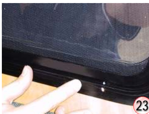
Line up holes in clamping with Mainframe
