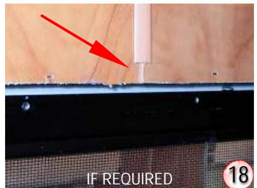
Top of window. T-section cut out the same height as the clampring. IF REQUIRED
