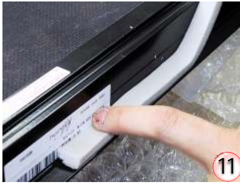
Clean dust and dirt from around the opening where the window is going to be fitted. Wipe window main frame flange with a dry cloth to remove dust. Apply bedding compound to flange. Foam tape is used in this case in the above picture.
