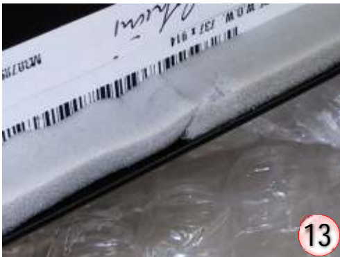
Apply foam tape all the way around the flange. Mid-Bottom of the window is a suitable starting point. Take particular care around the four radius corner. Cut off tape end at the starting point to form a continuous seal. Join foam tape, cleanly, as above. Apply bead of silicone to foam tape.
