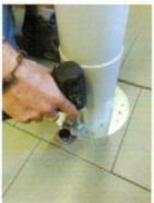
3 – Remove the plastic cover to expose the internal metal components
