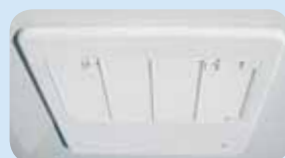
Ducted air intake grill
